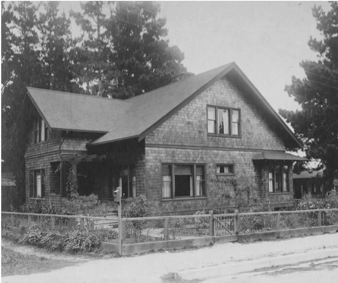
1918 SOUTH ELEVATION – 872 LAUREL AVE
