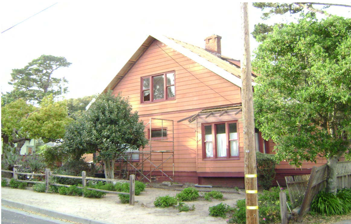
South Elevation with Aluminum Siding Installed in 1970s
